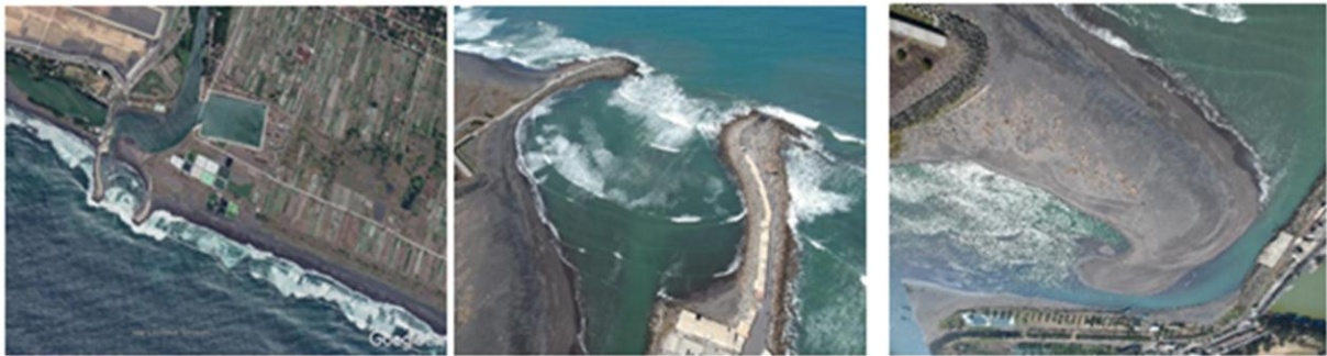
Figure 8. Condition of the Serang River Estuary blocked by sediment (Puspa et al. , 2020)
